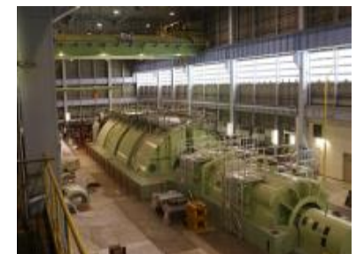
Tomatch-Atsuma Power Station
