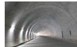
Coal ash is recycled into concrete used for tunnel linings.
